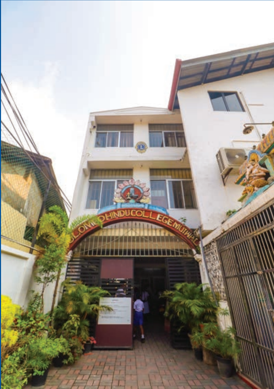
Project (08) Canopy constructed, at the School entrance completed and handed over STAGE 01
